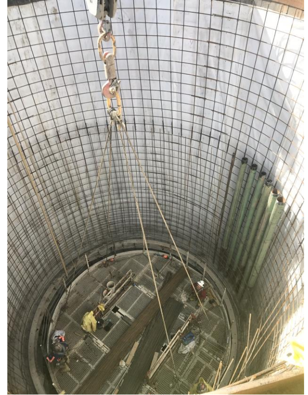
Shaft wall concrete preparations
